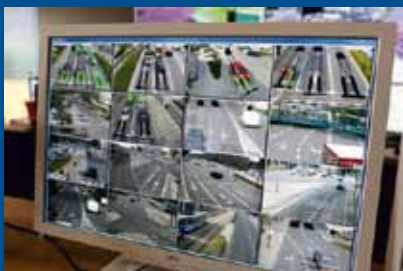
Monitor operatora podsystemu wideomonitoringu
